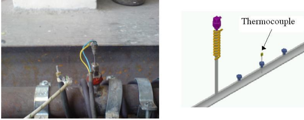
Figure 3.3 Thermocouple in drive section
